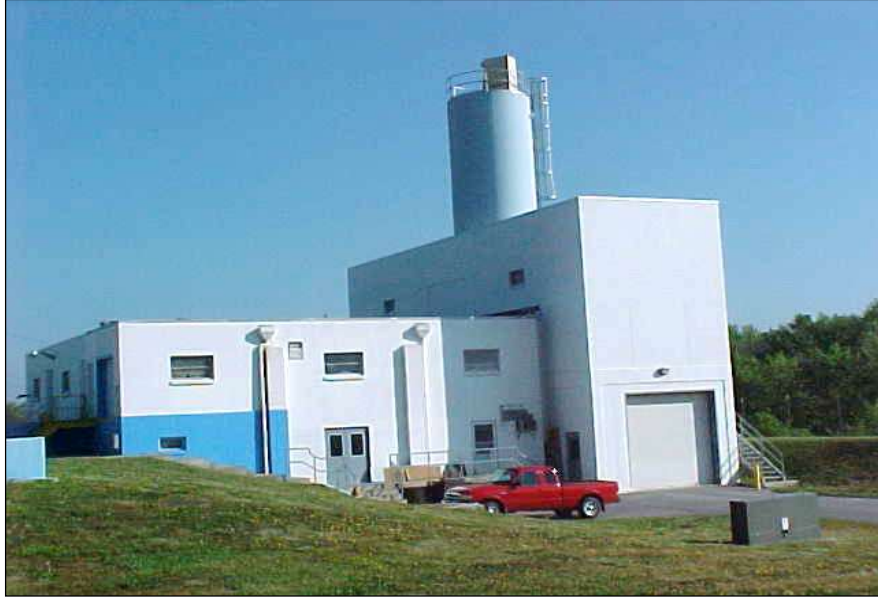
Filter building with lime silo
