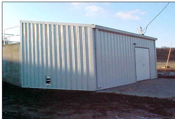
Effluent irrigation building
