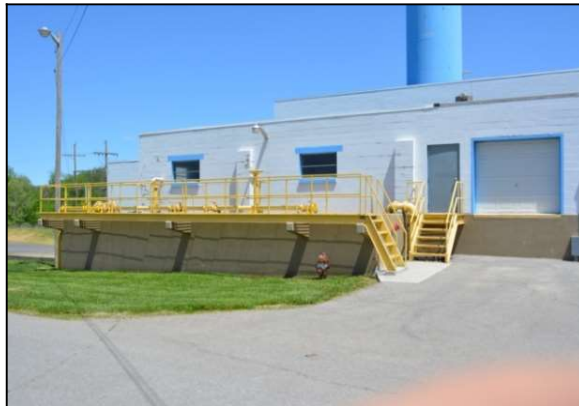
Waste sludge holding basin #1
