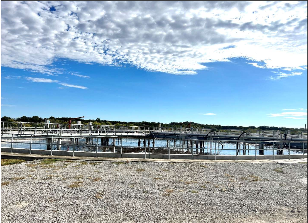
Upgraded Aeration Basin
