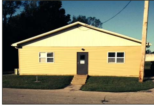
Office and laboratory building
