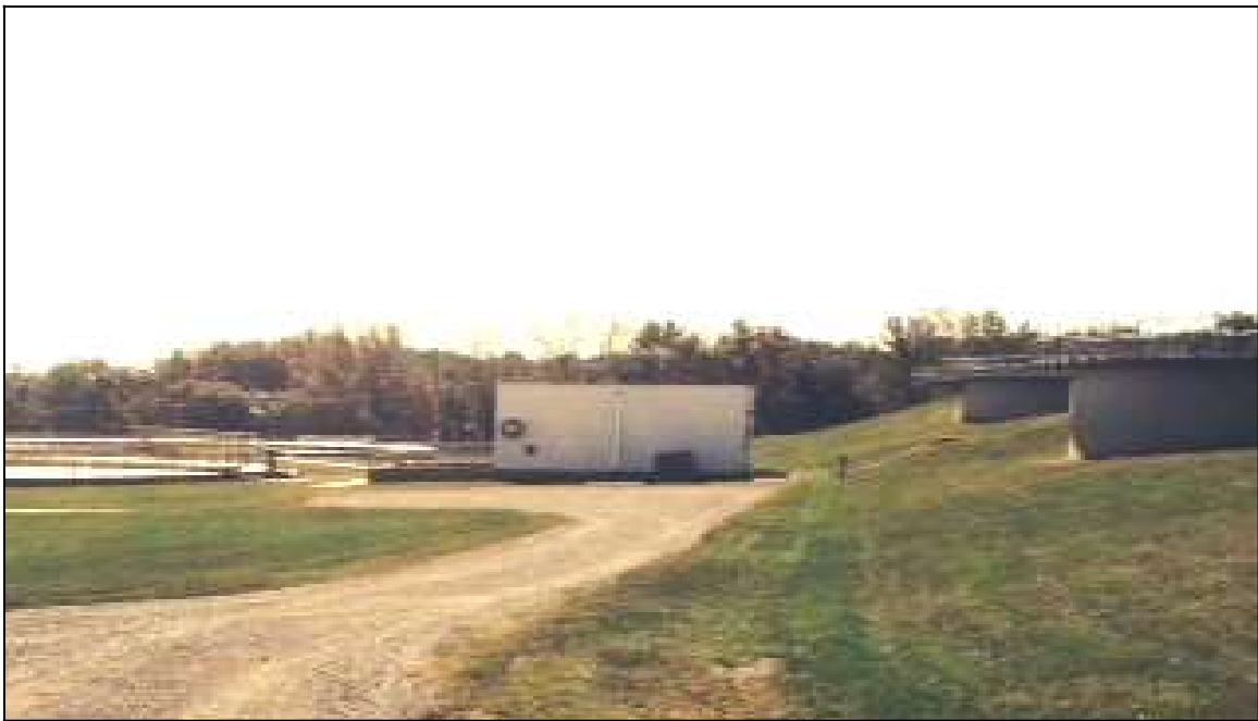
RAS building with final clarifiers to the left and aeration basins to the right
