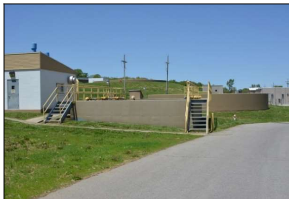
Waste sludge holding basin #2
