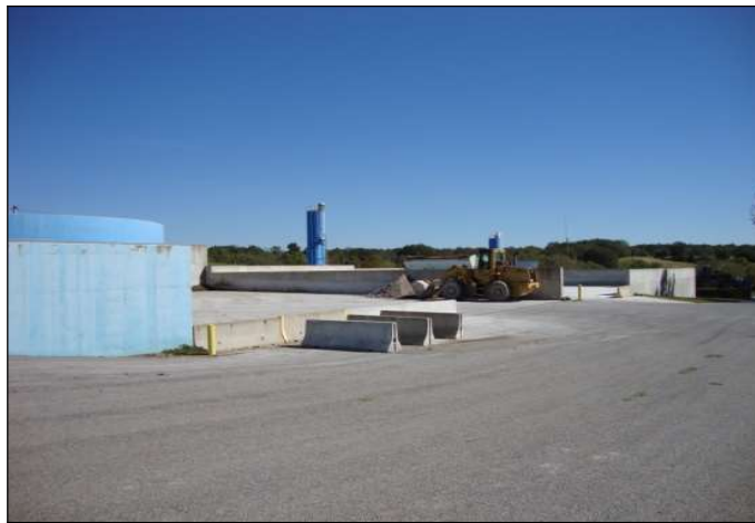
Sludge holding pads
