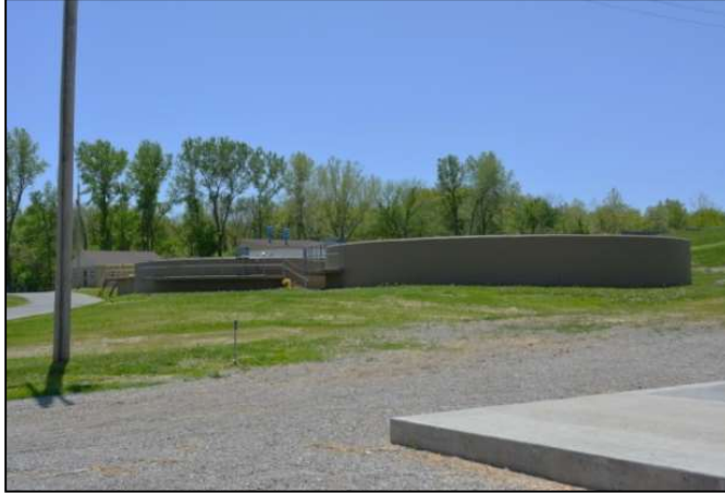
Waste sludge holding basins #3 and #4
