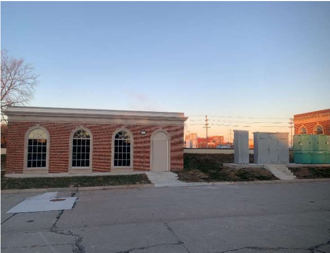
North Street Pumping Station 765 W. North Street
