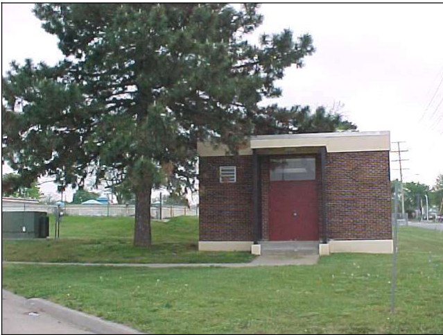
Miami Street Pumping Station
