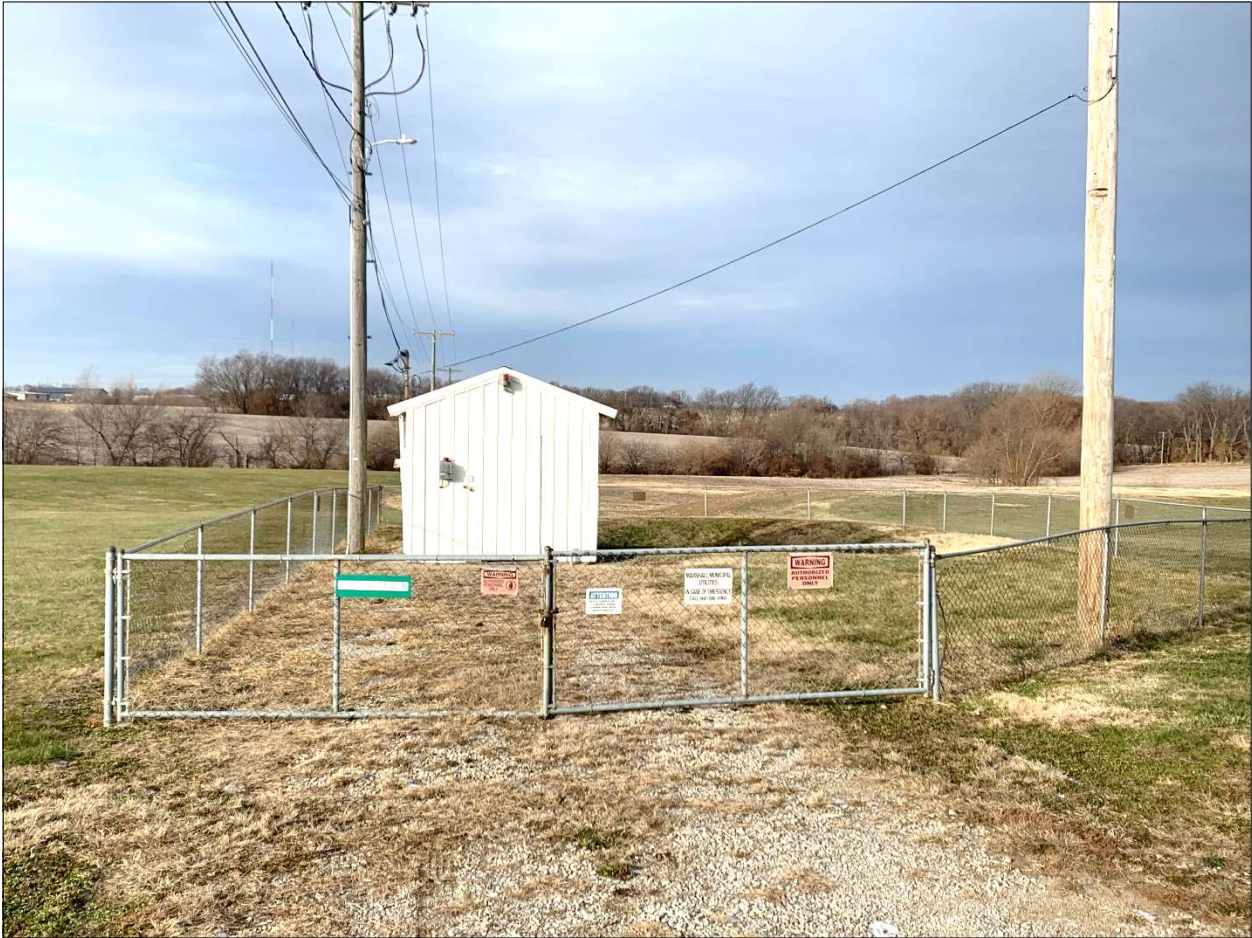
North Miami Sewer Lift Station North Miami and Darling Street
