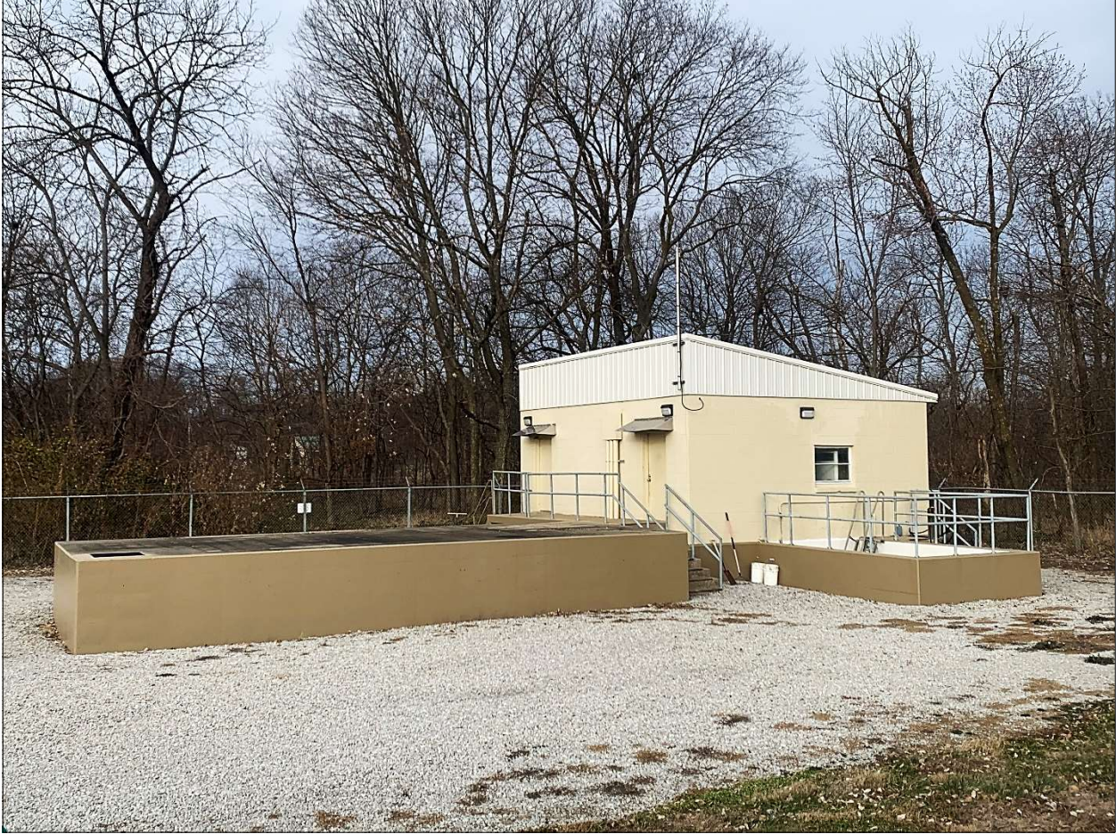
Southwest Sewer Lift Station Fairgrounds Road West of Hospital
