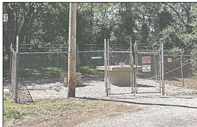
North Conway Sewer Lift Station
